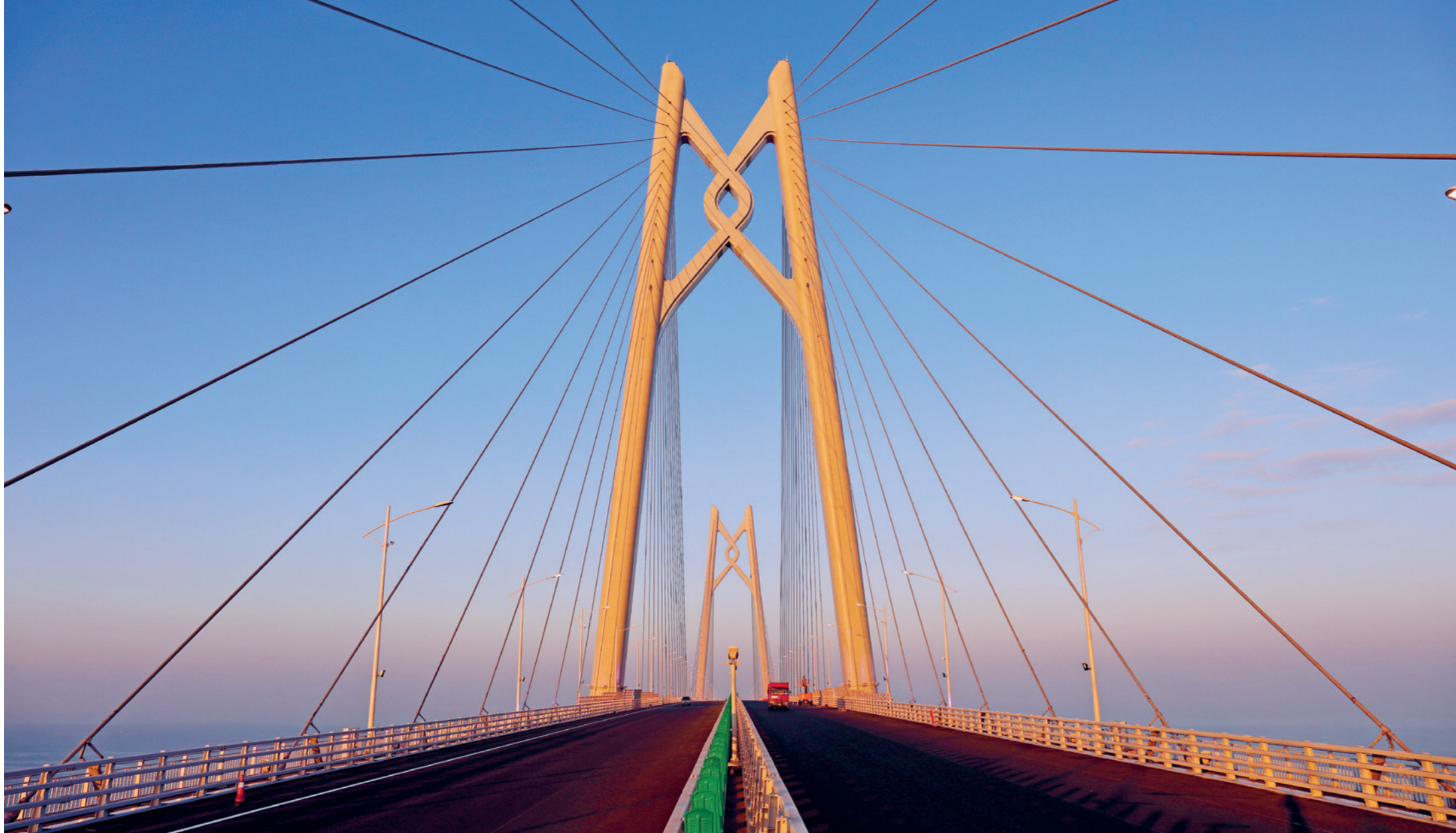
The Zhuhai section of the bridge links up Hong Kong and Macau in a 45-minute drive
