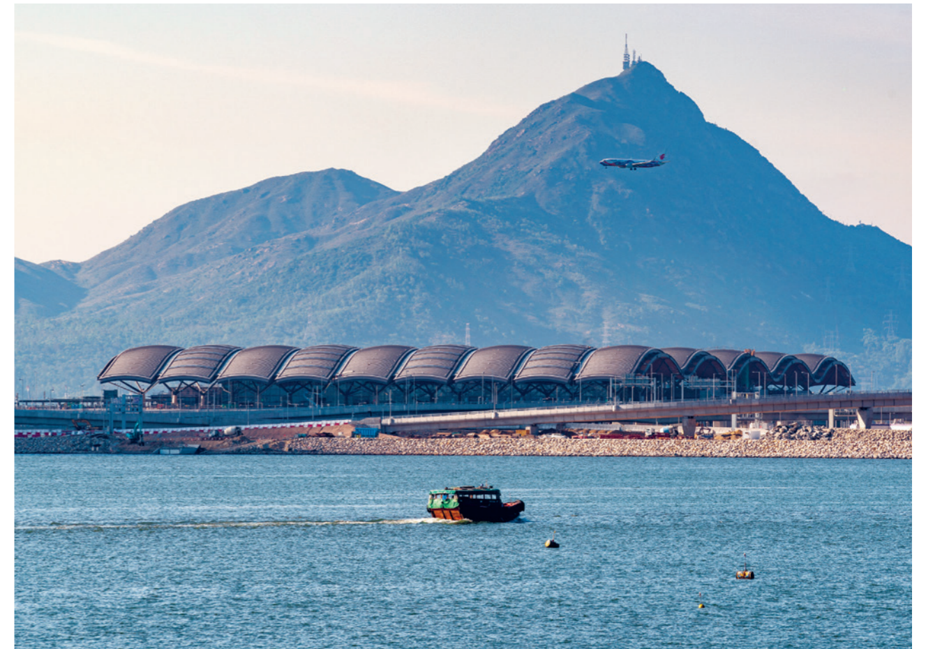
The Hong Kong-Zhuhai-Macao Bridge Hong Kong Port by Aedas and RSHP
